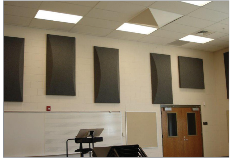
ESSI Barrel-Shaped Diffuser Panels used on walls
